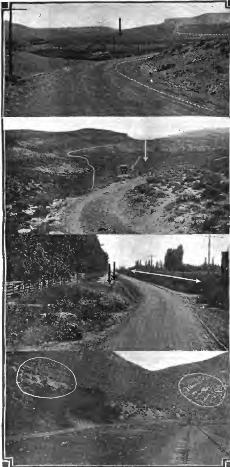
Top—A $40,000 shale and rock boulevard 15 miles long connecting Rock Springs and Green River, Wyo., winding its well-engineered way through one of the mountain ranges, west of the Rockies, in Wyoming. At each end is a town; between is not a habitation. The surrounding country is wild. Dotted line shows part of the old trail across the alkali bottom. Upper Middle—West of Green River, at the west end of the boulevard, shown in (M), the road is bad only by comparison. The soil is of the same type, largely gravel, shale and rock. Arrow shows road across alkali bottom. Line shows good bench for a road. Lower Middle—The importance of Salt Lake City and Ogden, and the value of the land between has brought about definite road construction, connecting the two, on modern lines. In the meantime the roadway yet to be completed by the engineers is in a generally excellent condition, although in places liable to have standing water because of high sides at certain points. White arrow is wide irrigation ditch. Black arrows show ruts indicating true character of soil. Bottom—The canyons that lead into Utah from the east are narrow winding valleys. The soil is all that could be desired for the construction of roads. Even now the little attention that has been given has yielded a roadway that affords excellent touring, there being considerable rock and a lot of surface gravel that rapidly shape themselves under the minimum of attention. Circles indicate mountain sides of rock and gravel.
